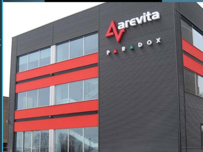
Каунас Paradox Distribution Centre
